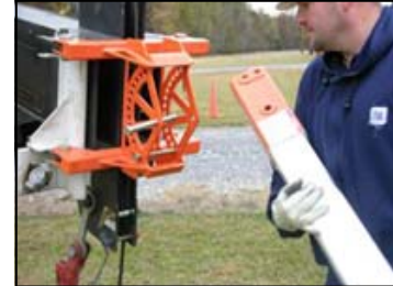
Installation of Jib
